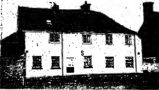
No 16 High Street, Langstone, on the foreshore of Chichester harbour
